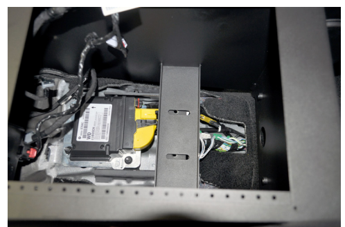
Reroute all OEM wires and reconnect.
